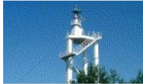
e.m. monitoring antenna
